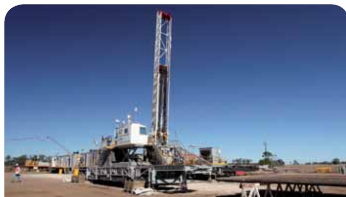
Installation of a trial aquifer reinjection bore
