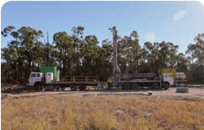
Installation of one of Australia Pacific LNG's many new monitoring bores
