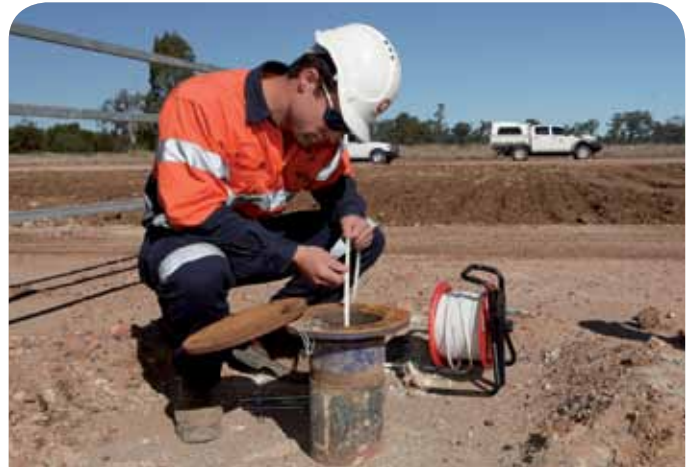
Measuring water levels in a monitoring bore
